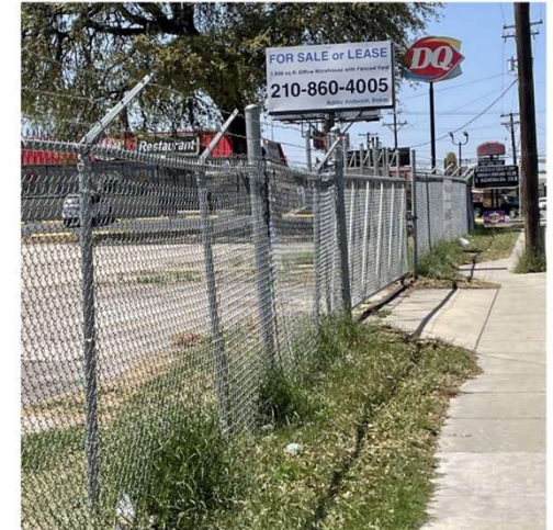
Site I* – Chain Link Fence
